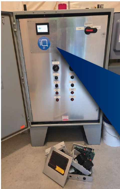
Before and after images of the lift station panel. Below showing the Horner X4R in the iQ2 Platform
