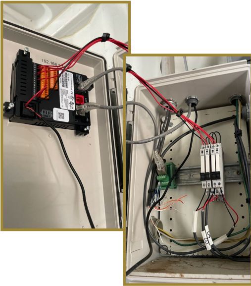
Current panel with Micro X4A
