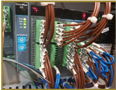
Horner SmartRail I/O in system
